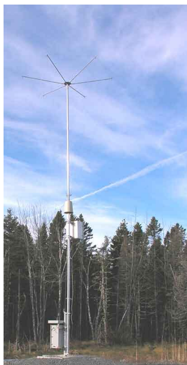
Nautel Cardinal CL-40 Antenna Systems
